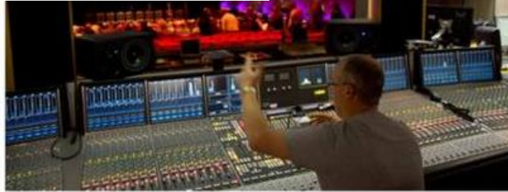
Theatre Control Room
